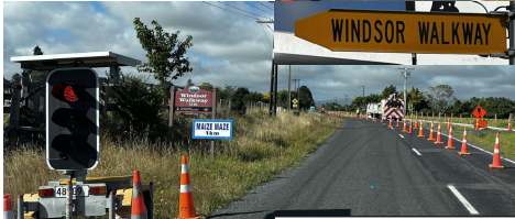
Above: Work starting on the Windsor Walkway
