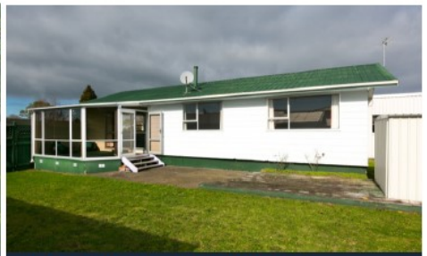
INGLEWOOD 7 Pokaka Place
